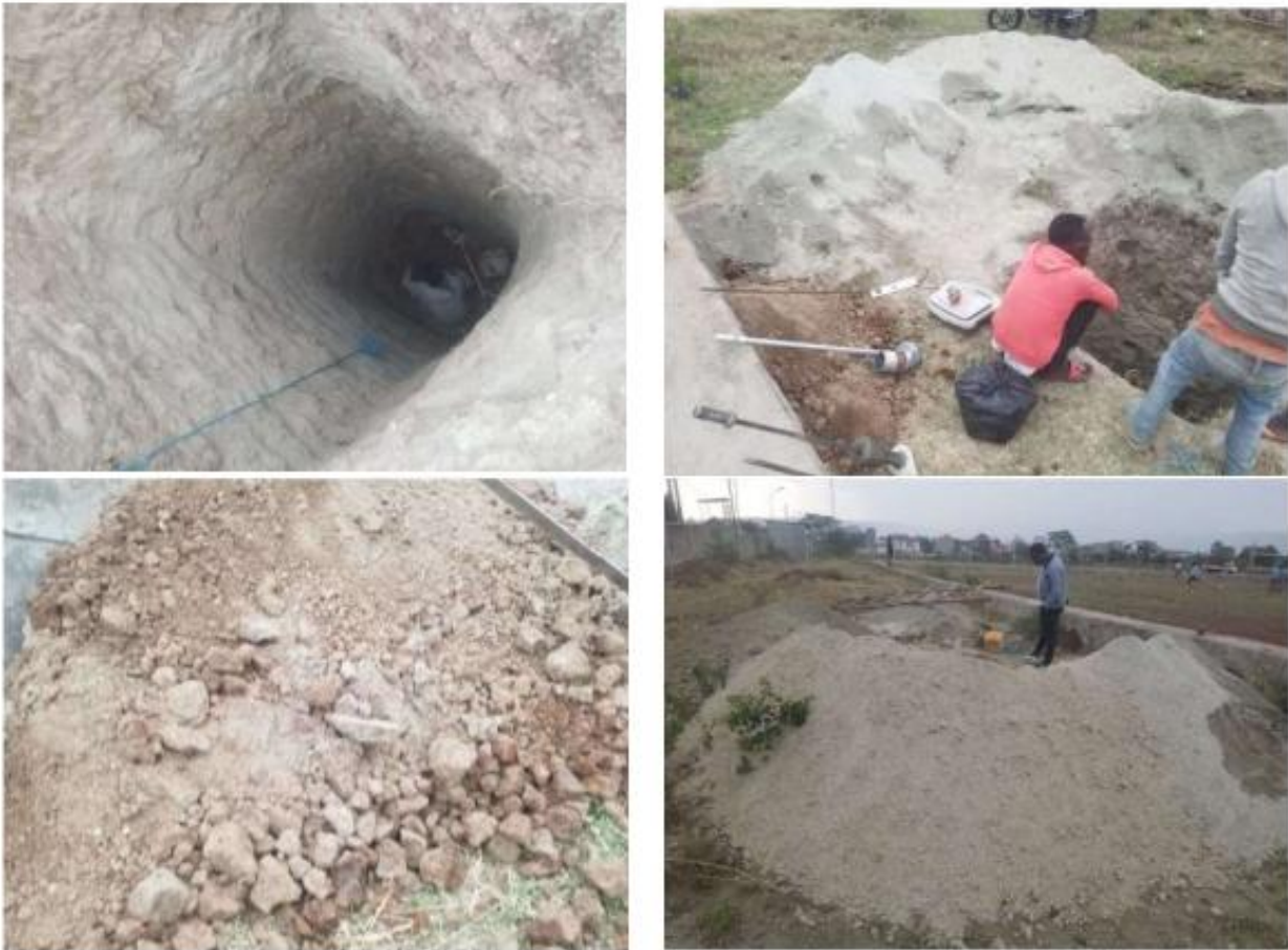
Figure 5. Partial Scene sat pit excavation site
