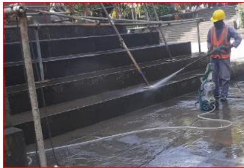
B) cleaning work on external staircase
