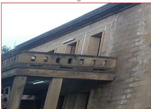
A) Efflorescence effect on the surface of the wall
