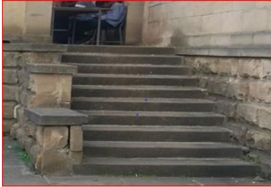
A) Deteriorated Steps of the building
