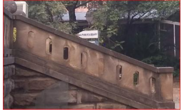
B) Deteriorated guard wall
