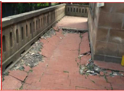
B) damaged tiles, floor finish on verandas
