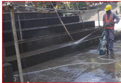
B) cleaning work on external staircase
