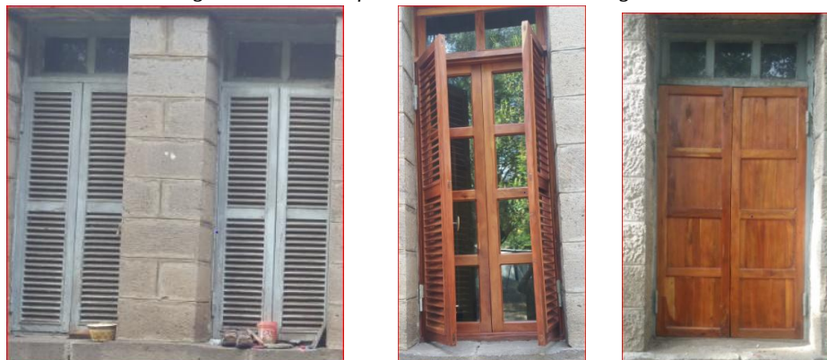
A) Deteriorated window frames B) Windows of the building after maintenance
