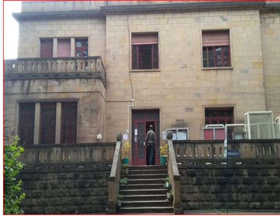
A) Front view of the building
