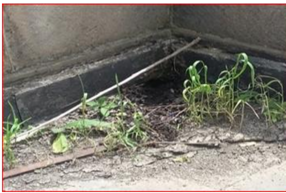
A) Growth of plants on the roof slab
