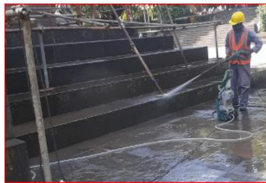
B) cleaning work on external staircase
