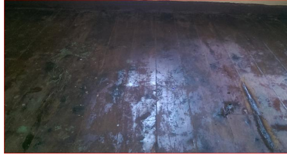
B) Well-maintained floor finish
