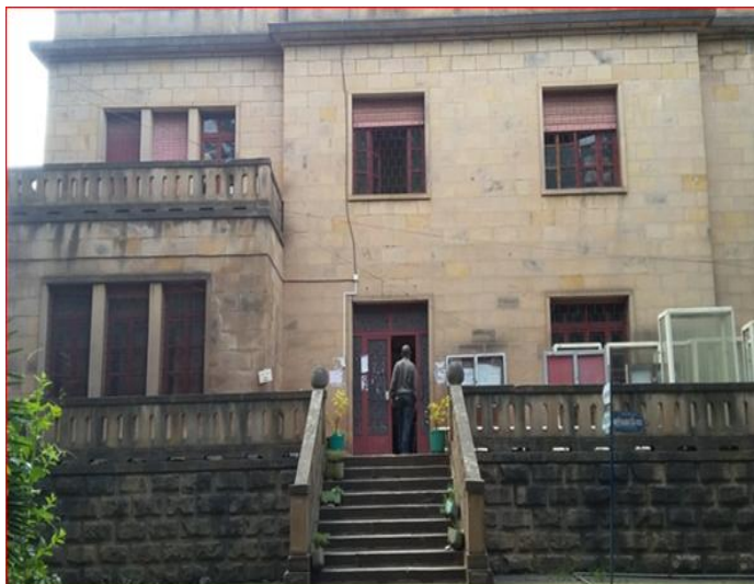
A) Front view of the building
