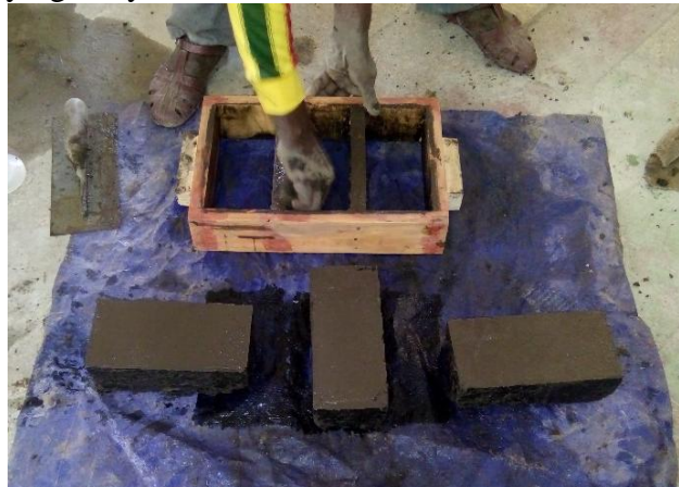
Figure 3. Mold used for casting adobe bricks
