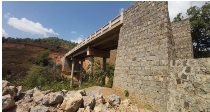
Figure 2 Partial View of Logita Bridge, abutment and approach embankment retaining wall under construction
